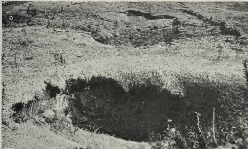
FIG. 20.—Detail of a cave on a hillside near Streator; note the hanging sod.
